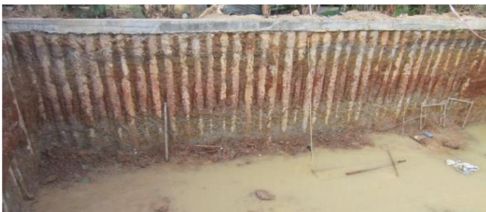
**Fig 3. Stabilization of diaphragm wall by bored pile D300.**
