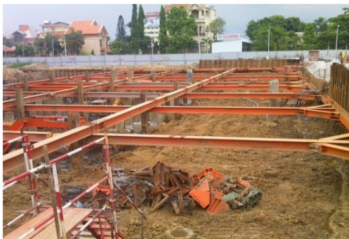
Fig 2. Shoring system combined with Larsen sheet wall.
